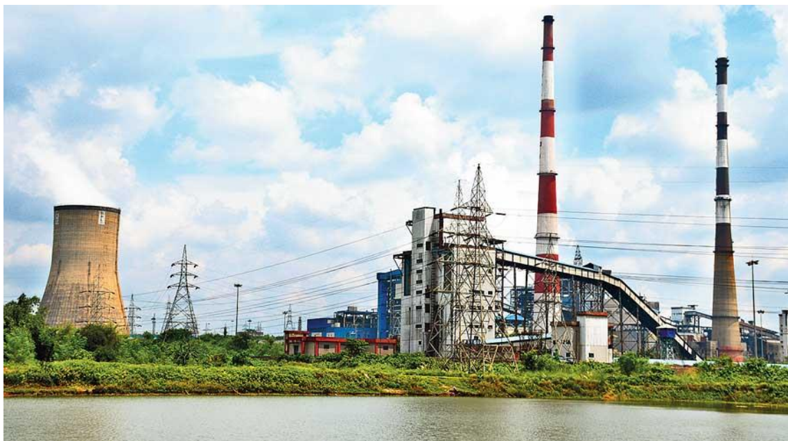
Photo: Duragapur Project Limited, Source by Internet
